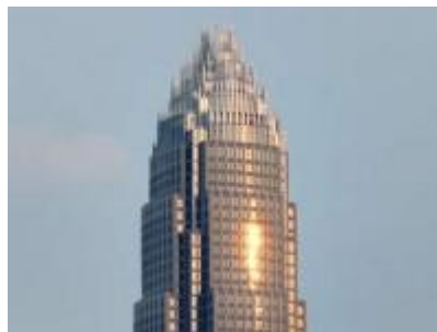
Tower Bank of America
